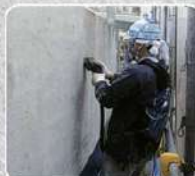
Clean to prepare the concrete surface.
