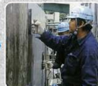
Apply binding solution.
