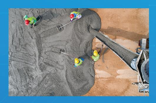
Ready-mixed concrete has a compressive strength range of 180-400 kg/sq.m., making it appropriate for general structures such as beams, poles, and floor bases.
